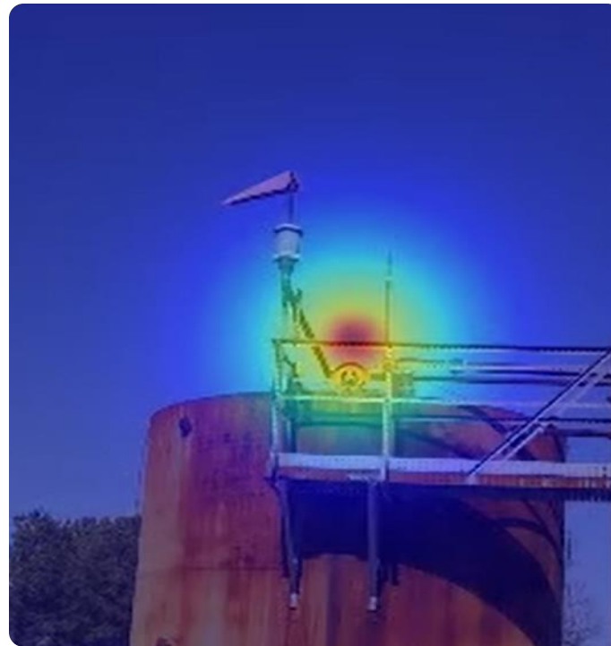
Emission on tank from the ground
